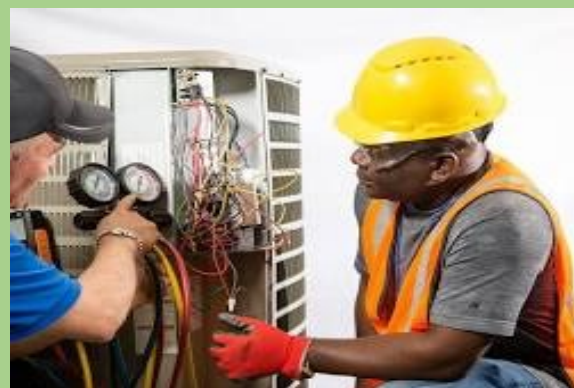
HVAC technician Heating, Ventilation and Air Conditioning)
